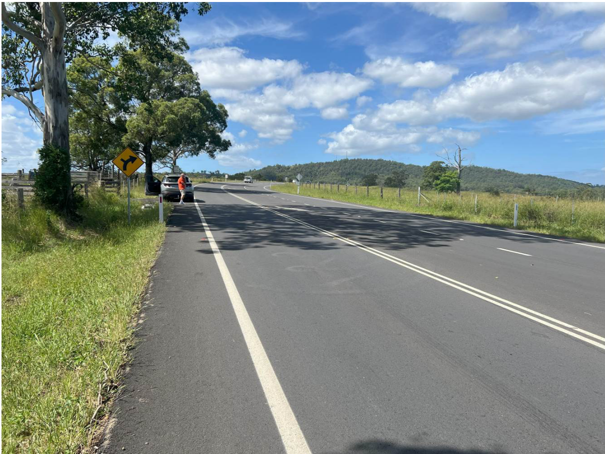
Photograph 4 – Wingham Road near existing site access
